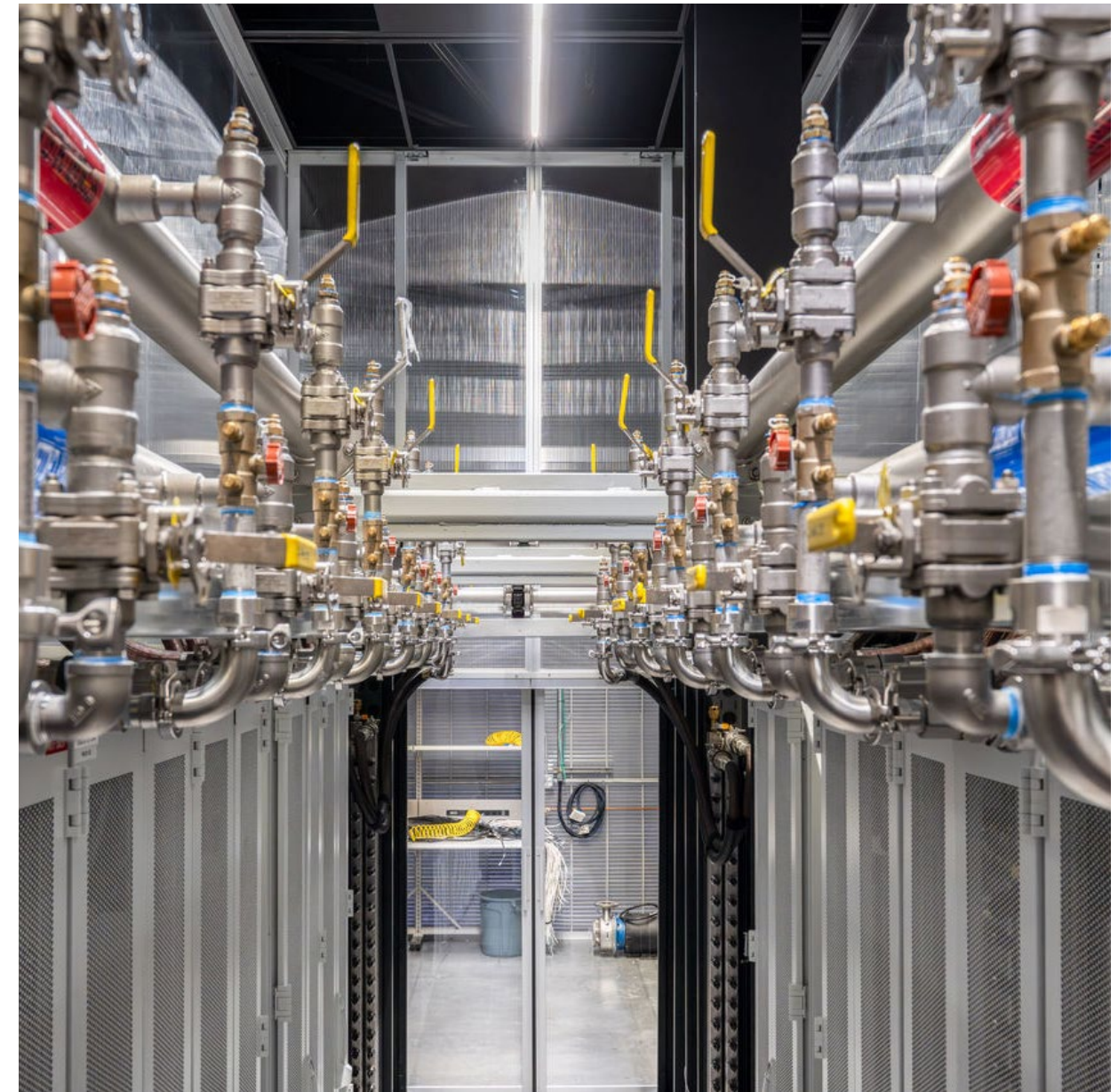
Equinix high-density liquid cooling infrastructure.
